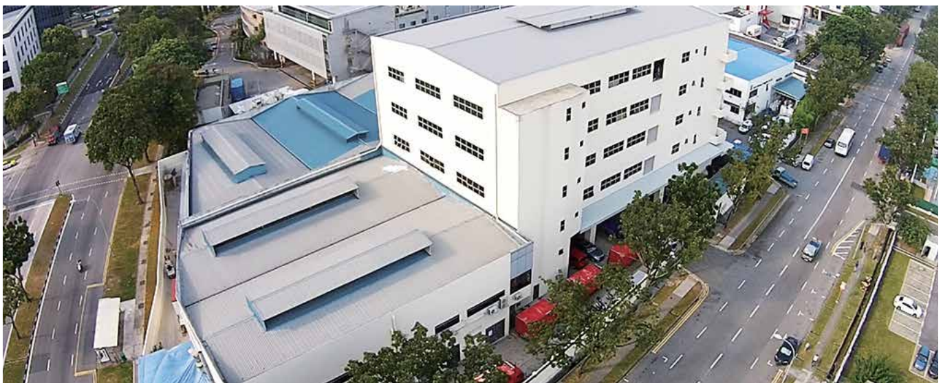
Our modern food manufacturing facilities at 30 Senoko South Road Singapore 758088
